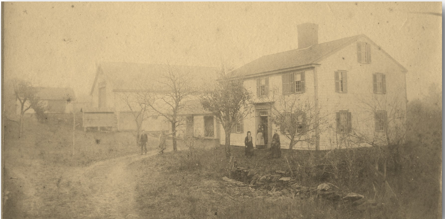
Early view of Haselton Barn, without cupola, and adjacent house
