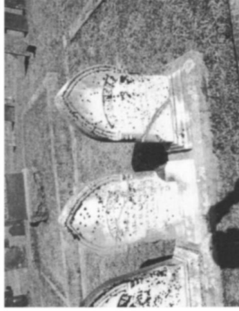
#11 — Headstone of Cordelia Chase [Blodgett-74], (sitting loose on base, needs to be refastened (center). Disposition: to be remounted by contractor (probably needs new pins plus cement).
