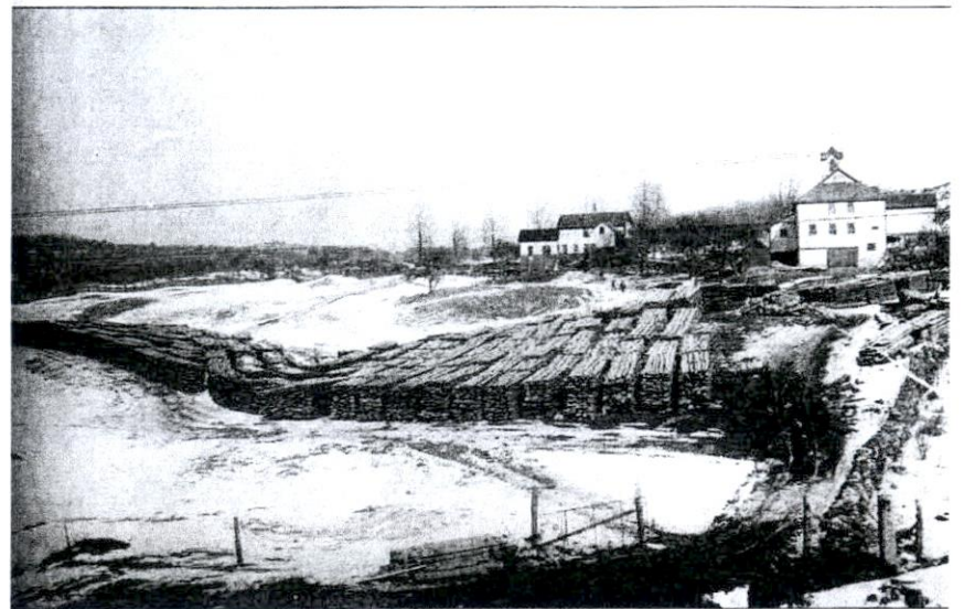
This is a view of the rear of the Haselton barn on Bush Hill Road.
