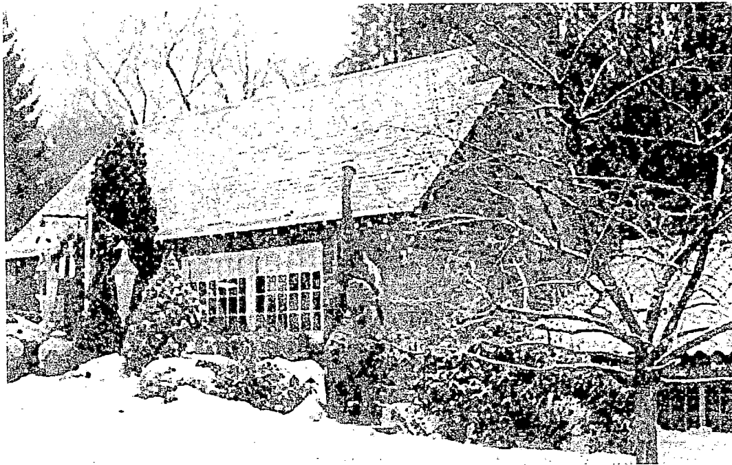
Figure 2. Benson's Office from the southwest. Date unknown. Used with permission of Robert J. Goldsack.
