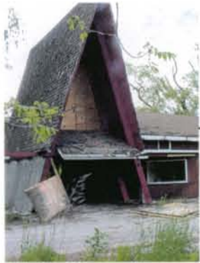
Existing Concession Building
