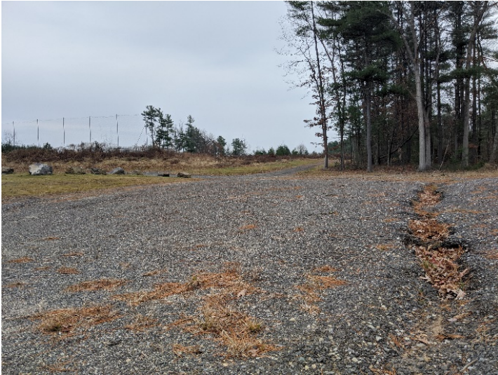
Photo 2: Visible erosion from flow concentration
