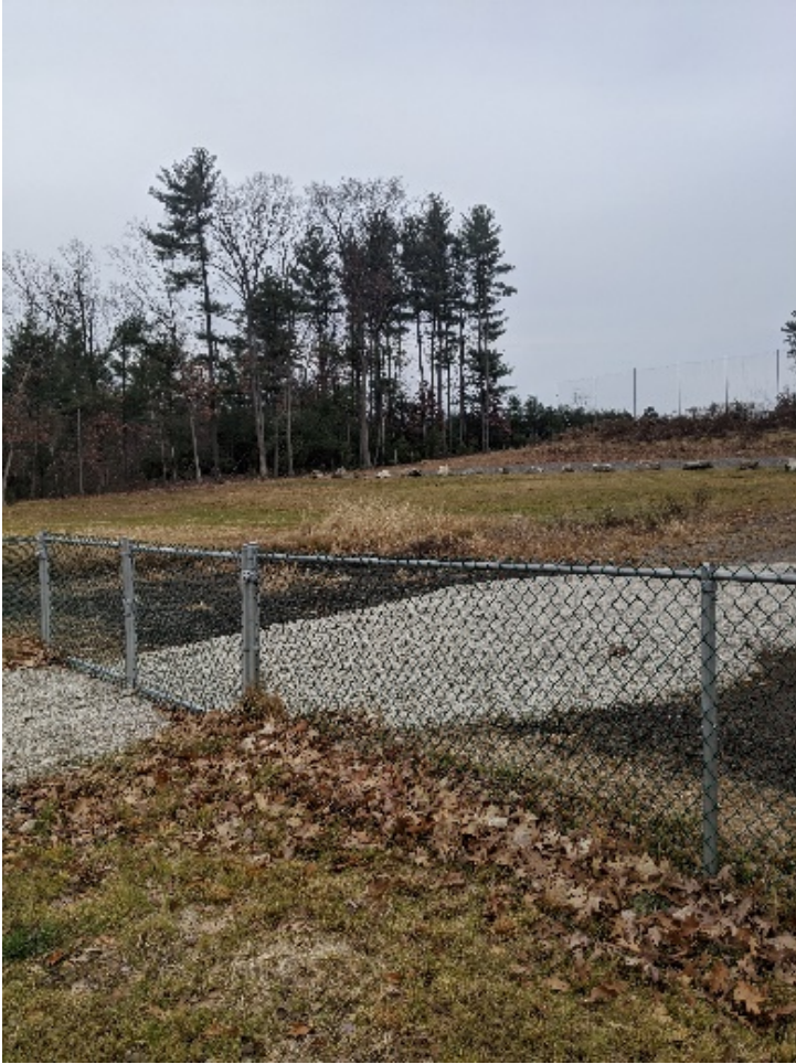
Photo 1: Drainage to depressed area. Looking northeast from the gate to the field
