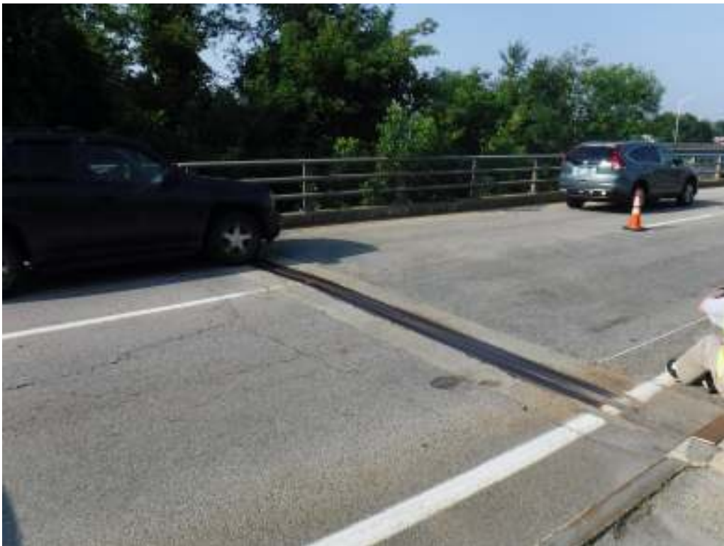
Photo 4 – Approach roadway looking west
