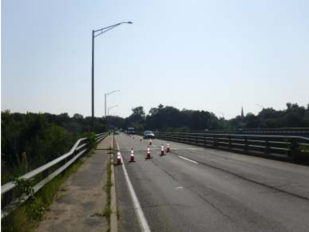
Photo 3 – Approach roadway looking east
