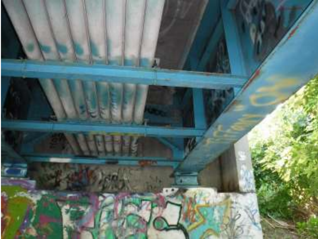
Photo 17 – View showing typical girder end conditions at the east abutment
