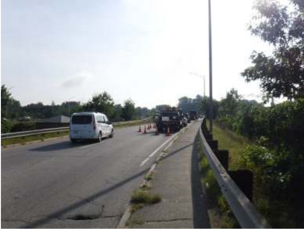
Photo 3 – Approach roadway looking east
