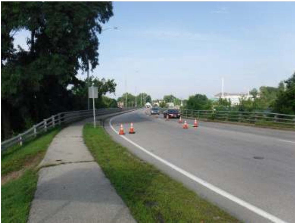
Photo 4 – Approach roadway looking west
