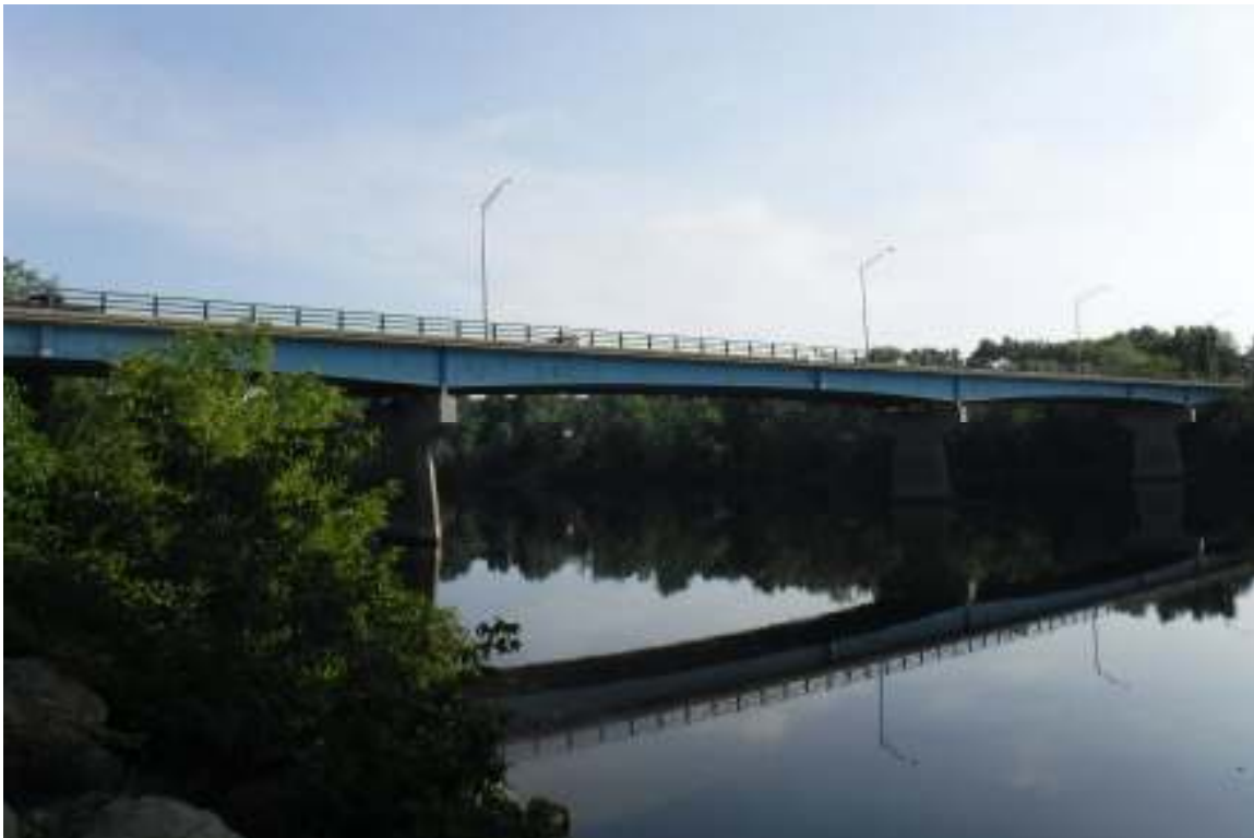
Photo 2 – Elevation view looking north
