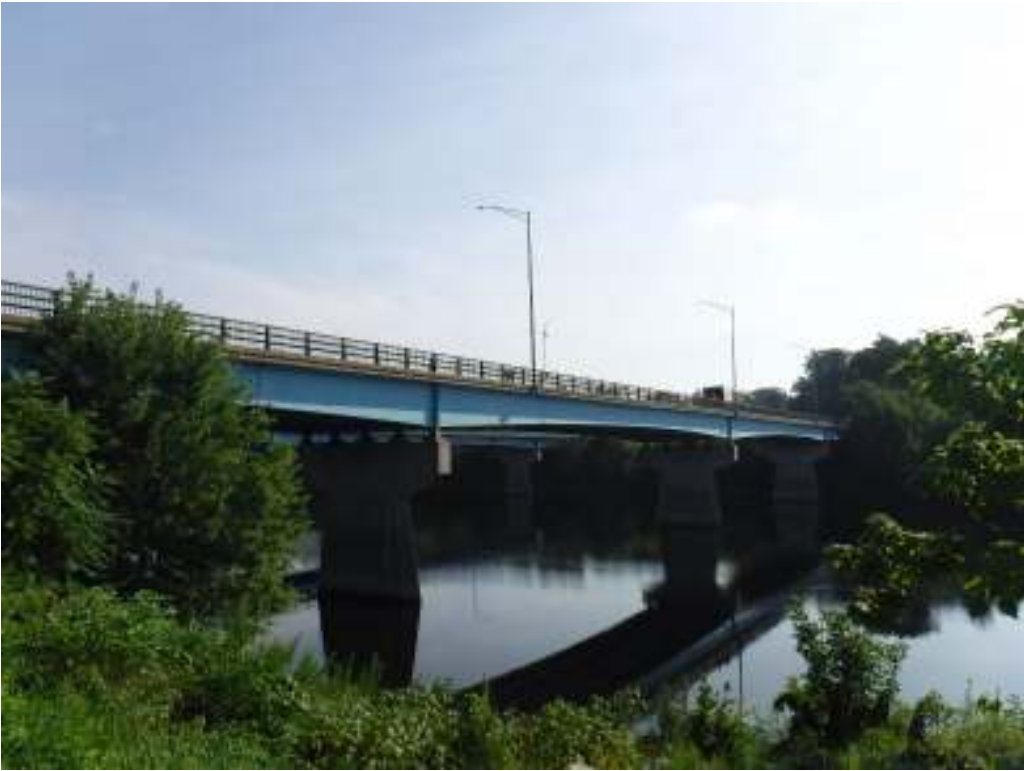
Photo 2 – Elevation view looking north
