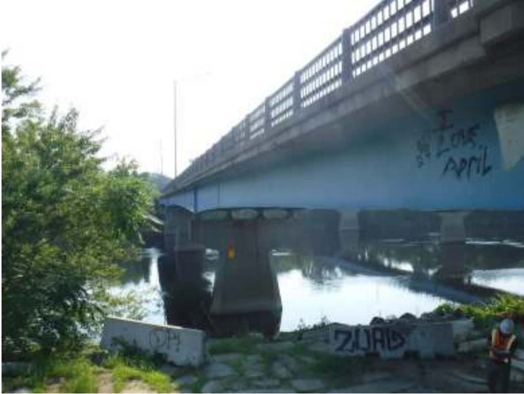
Photo 1 – Elevation view looking south
