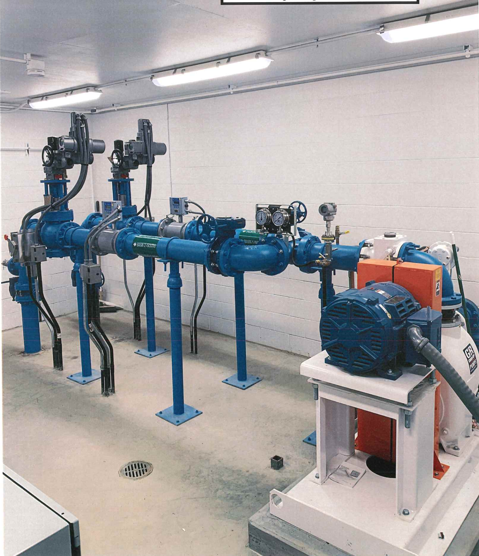
Dover, NH - Bellamy Recharge Facility Pump & Pipe Installation
