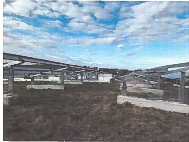
Racking structures installed on ballast blocks
