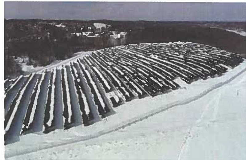
Ballasted fence installed and wiring completed
