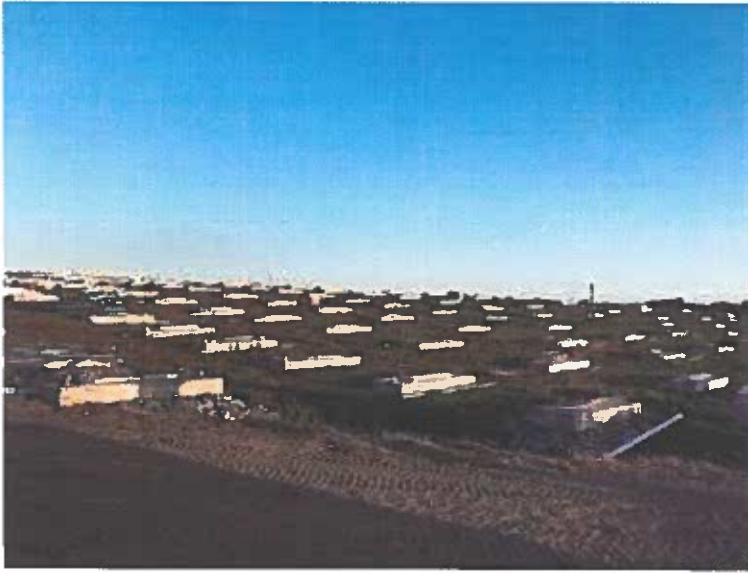
Ballast Blocks placed on landfill cap
