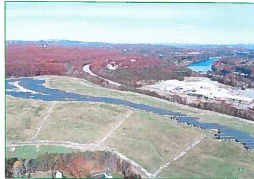
3.3 MW Kearsarge Manchester (Manchester, NH)
