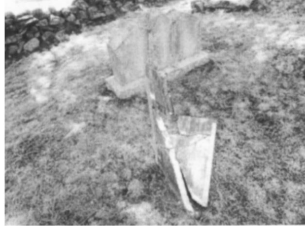
#19 — Broken headstone of Lucy Greely [Senter-8], wife of Alfred Greely, top of hill. Disposition: needs to be repaired by contractor.
