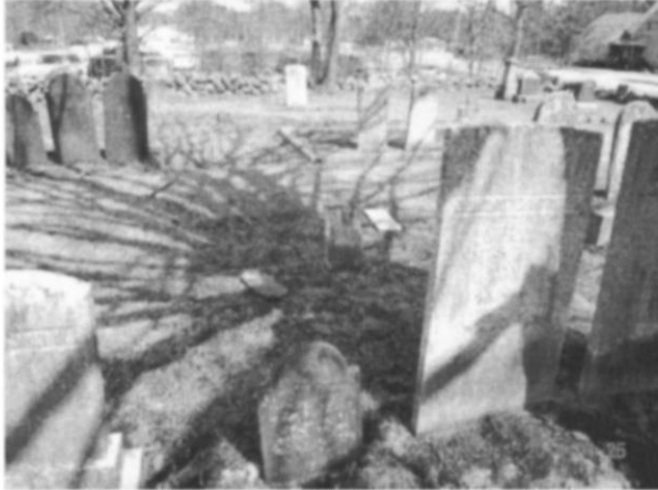
#7 — Fallen footstones behind headstones of Ann & James Page [Blodgett-65] (either side of Charles Page). Disposition: trustees will reset.
