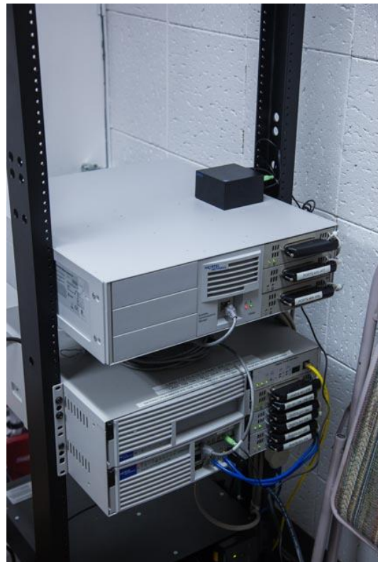
Town Hall and Police Nortel phone systems (BCM) in need of replacement FY16 and FY17.
