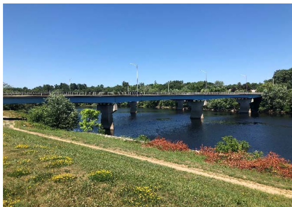
Taylor Falls/Veterans Memorial Bridge over the Merrimack River at the Nashua/Hudson Town Line
