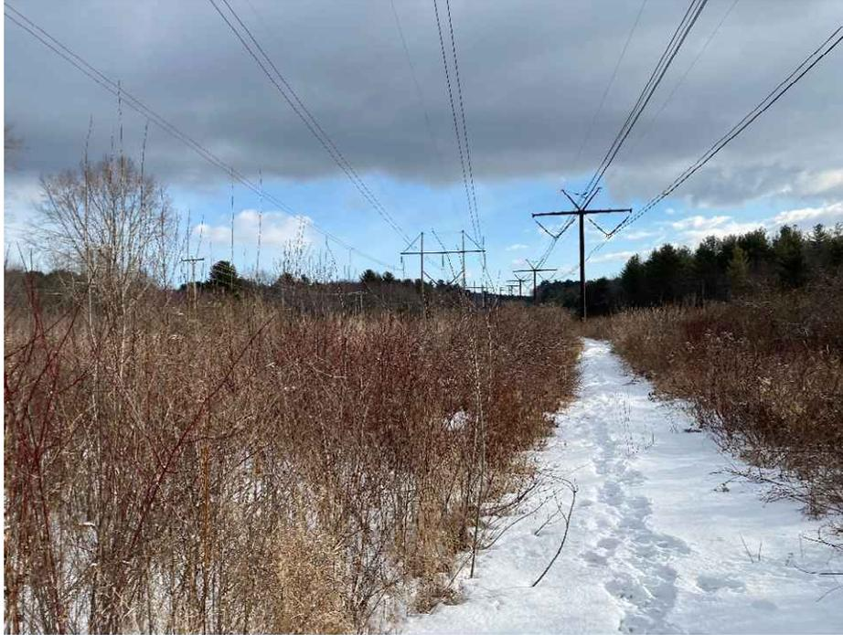
Photograph No. 3: Looking northeasterly at proposed access towards Structure 153 of the 326 Line to be replaced, across Wetland H-81. Timber matting will be used in the wetland portion of the access route.
