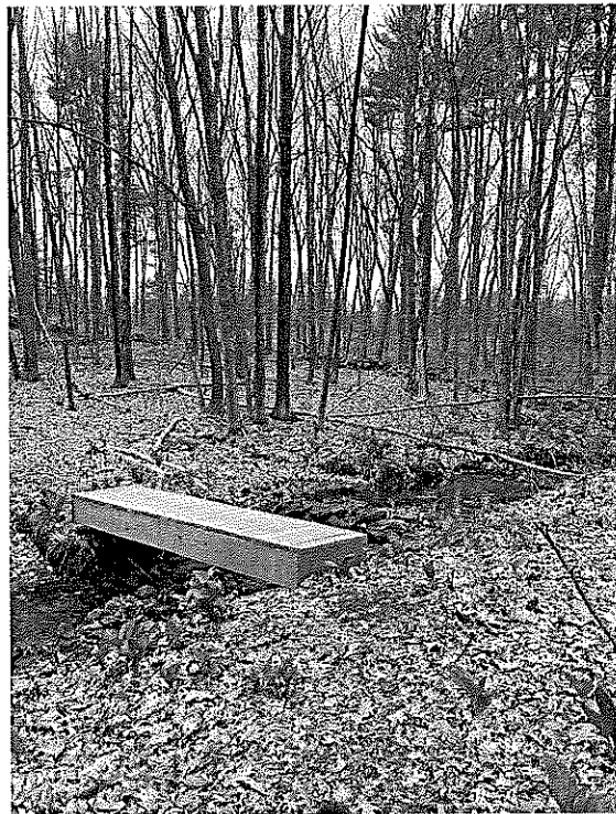
One of two new bridges installed by Boy Scouts in Nash parcel
