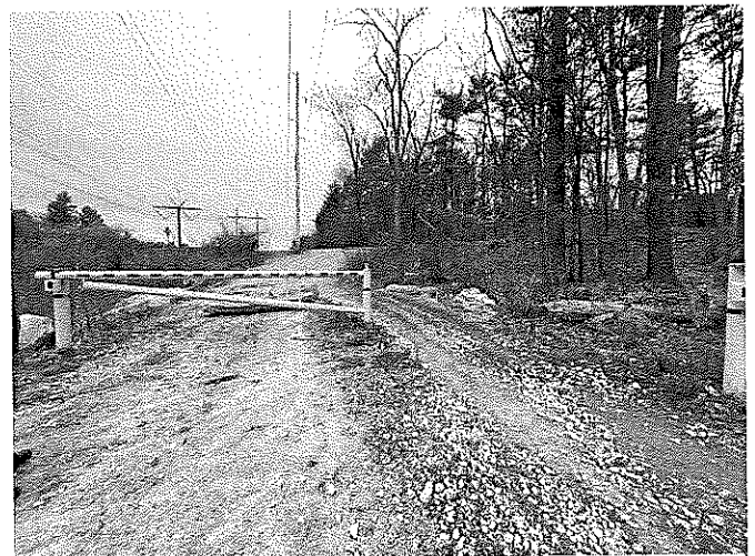
Gate at SW end of powerline ROW. Evidence of ATVs driving around gate.
