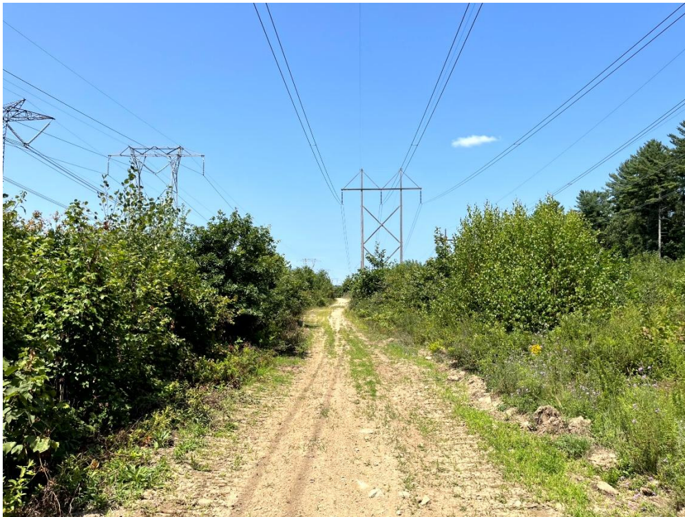
Photograph No. 1: Looking northwest at the proposed access road towards Structure 74 off Boyd Road, Hudson.
