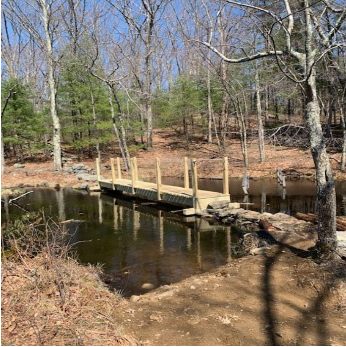
Photo 2: Newly constructed bridge near Second Swamp
