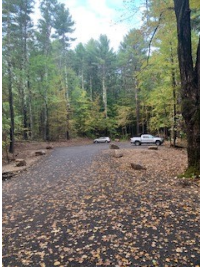
Photo 6: New parking area
