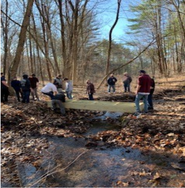
Photo 3: Newly constructed bridges, thank you BSA
