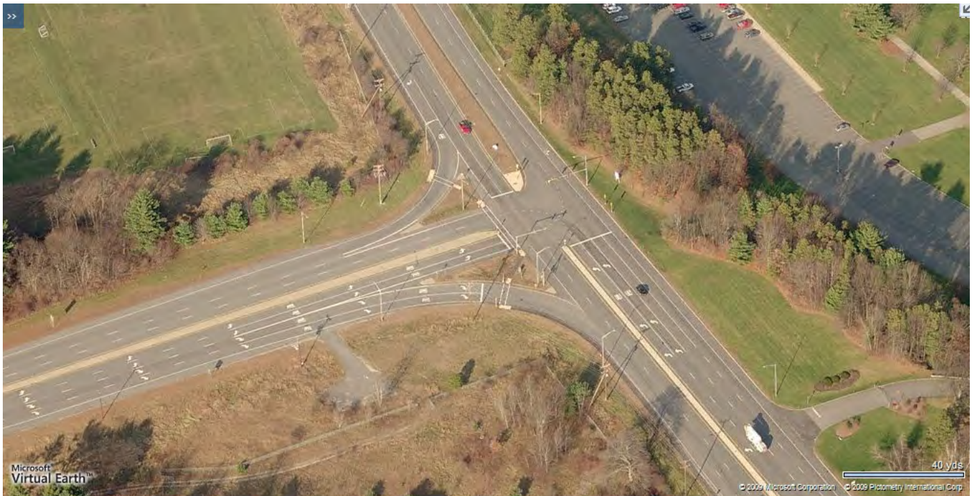
FIGURE 3: INDUSTRIAL DRIVE AND D.W. HIGHWAY/US 3 NEAR EXIT 10 IN MERRIMACK, NH
