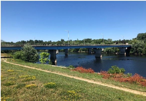
Taylor Falls/Veterans Memorial Bridge over the Merrimack River at the Nashua/Hudson Town Line
