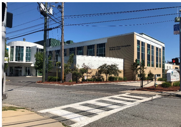
Southern NH Medical Center in Nashua relies on the Taylor Falls/Veterans Memorial Bridge for access to the region
