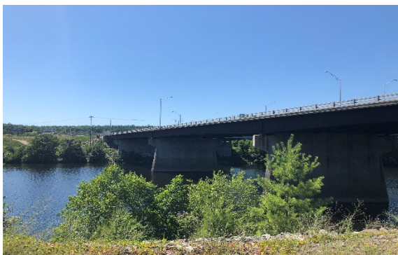
Sagamore Bridge over the Merrimack River at the Nashua/Hudson Town Line
