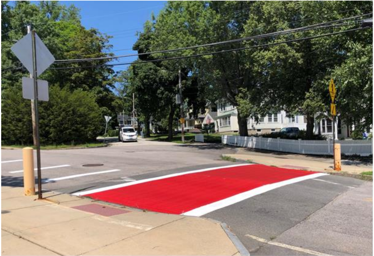
Raised Crosswalk in Nashua
