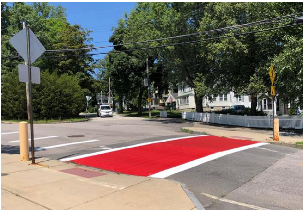
Raised Crosswalk in Nashua
