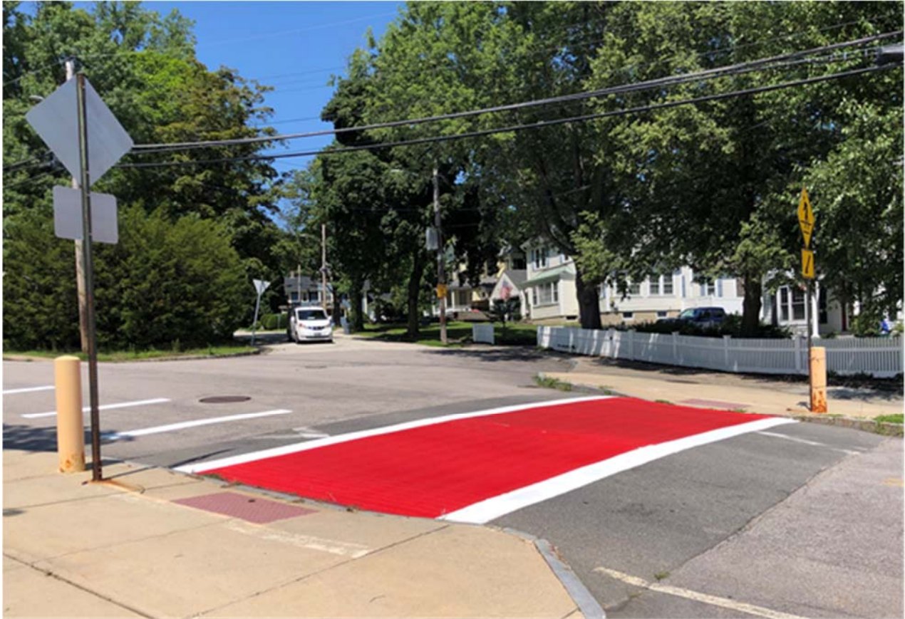
Raised Crosswalk in Nashua
