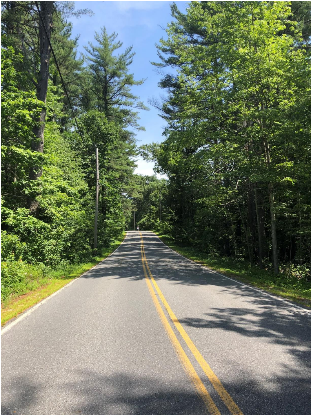
Wason Road, pictured above, has experienced high Levels of traffic growth
