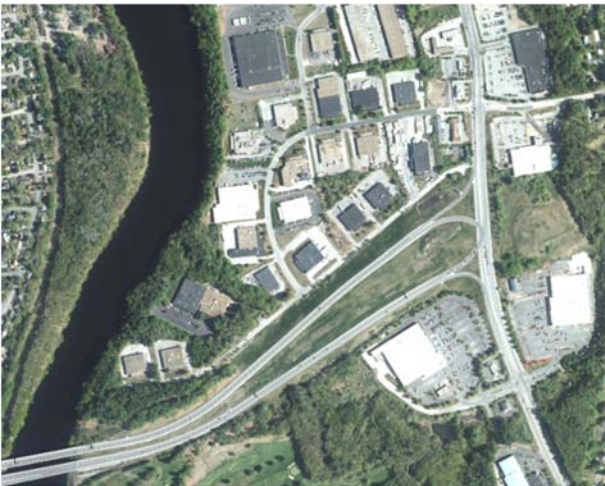
Above: Aerial Photo of Sagamore Bridge Area
