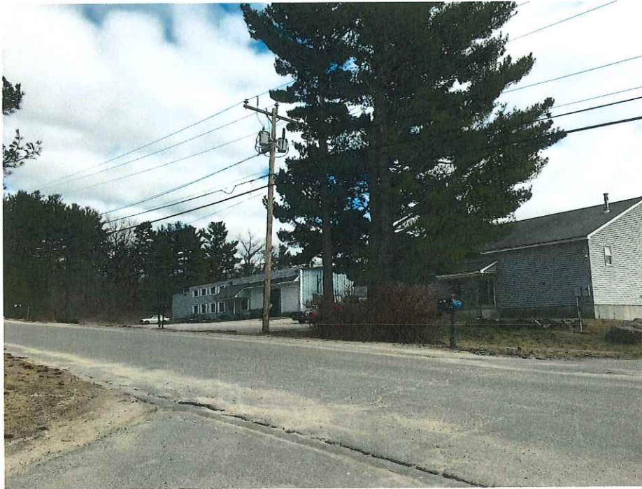
Photo No. 19: A view looking north easterly towards existing buildings to be razed.
