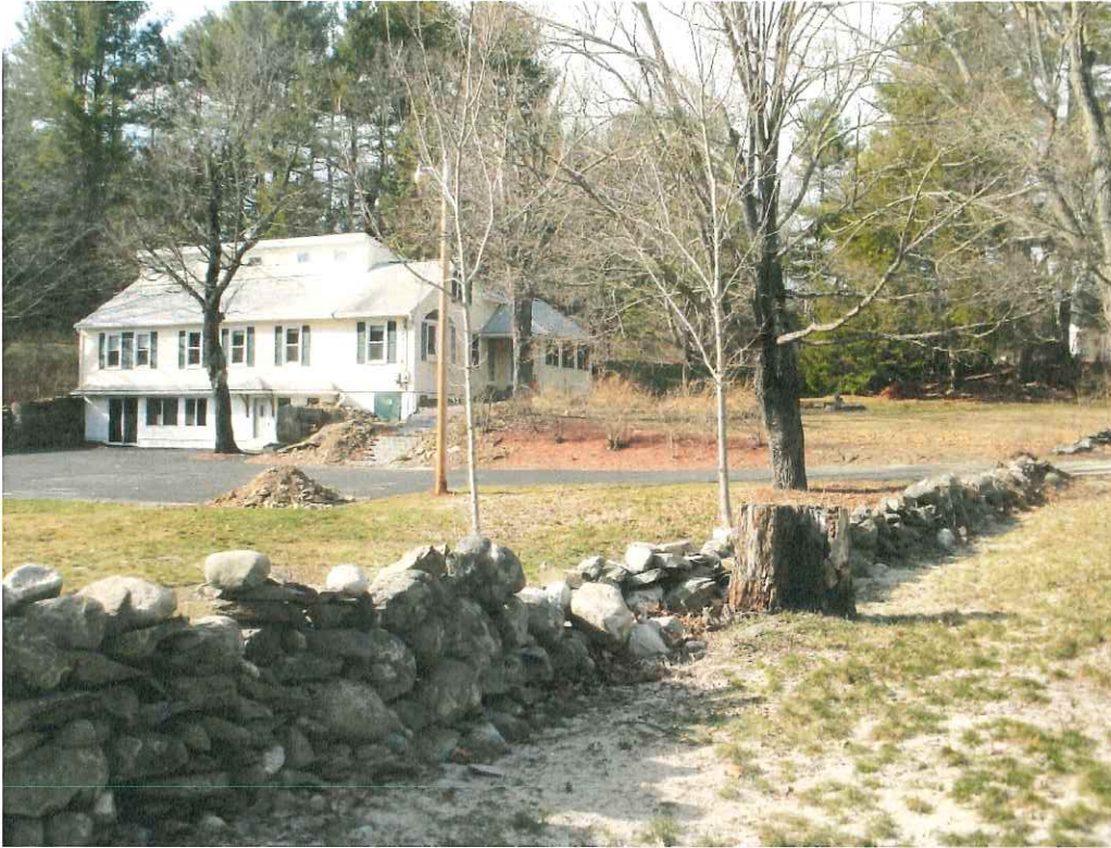
Looking north from Old Derry Road towards existing building
