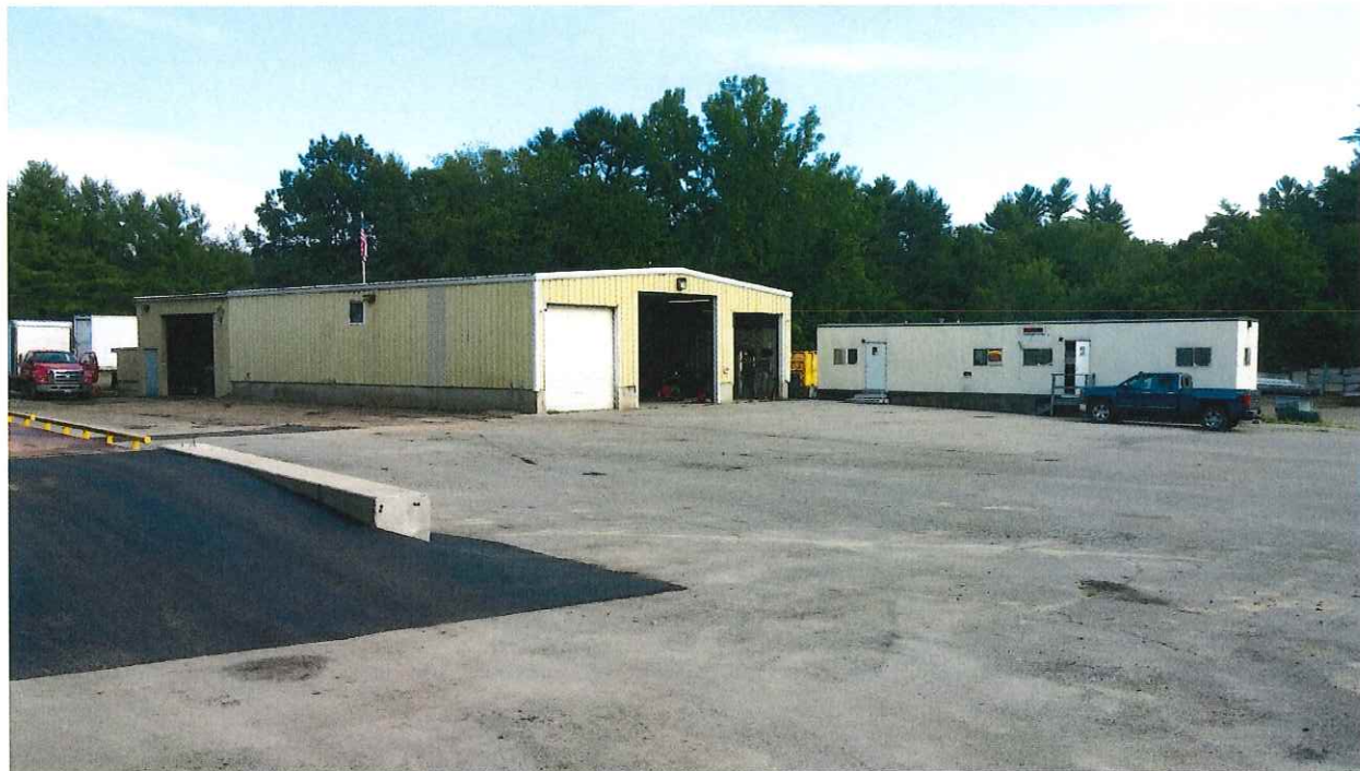
Photo#4 – The existing single story building and trailers, to remain
