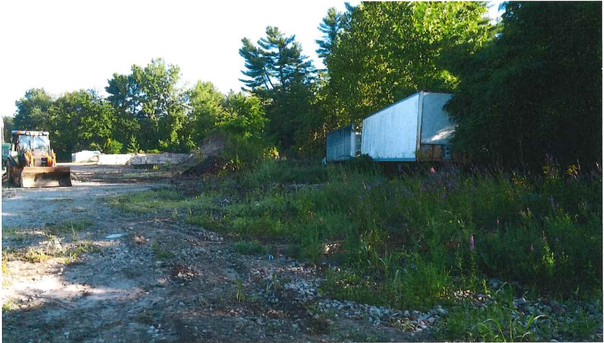
Photo #1 – Looking northwest at the existing site conditions (gravel surfaces, stockpiles, jersey barriers, equipment, etc.)
