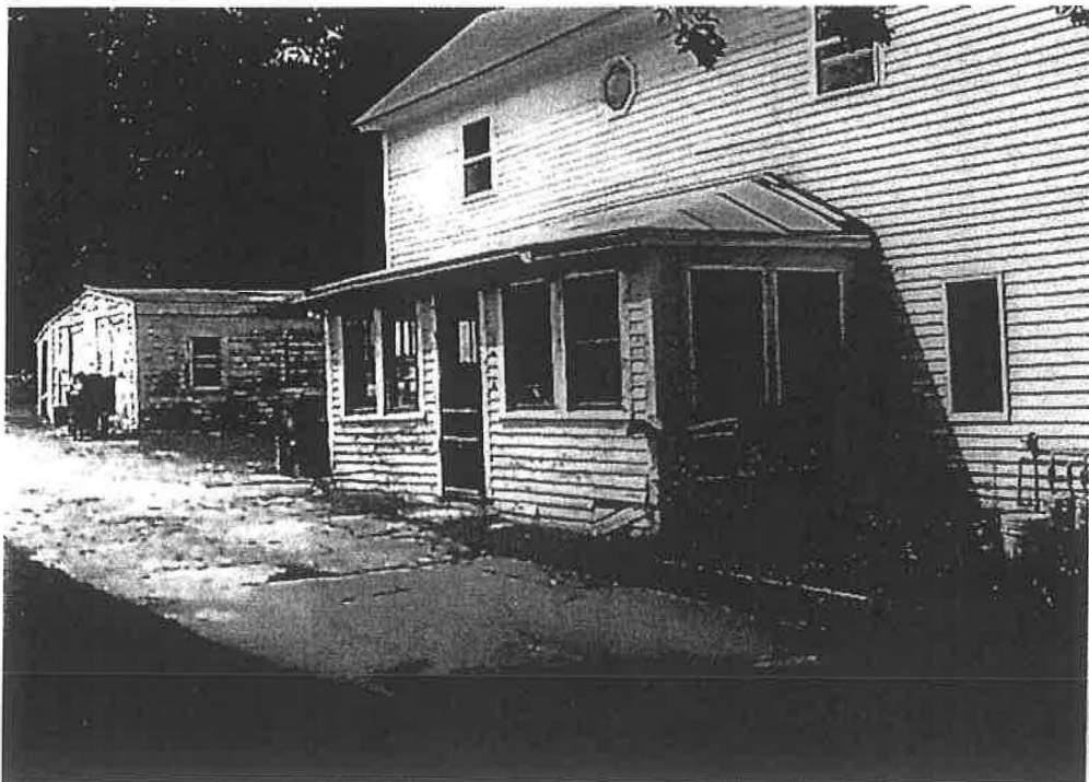
Photo No. 2: The existing two-story wood frame house.
