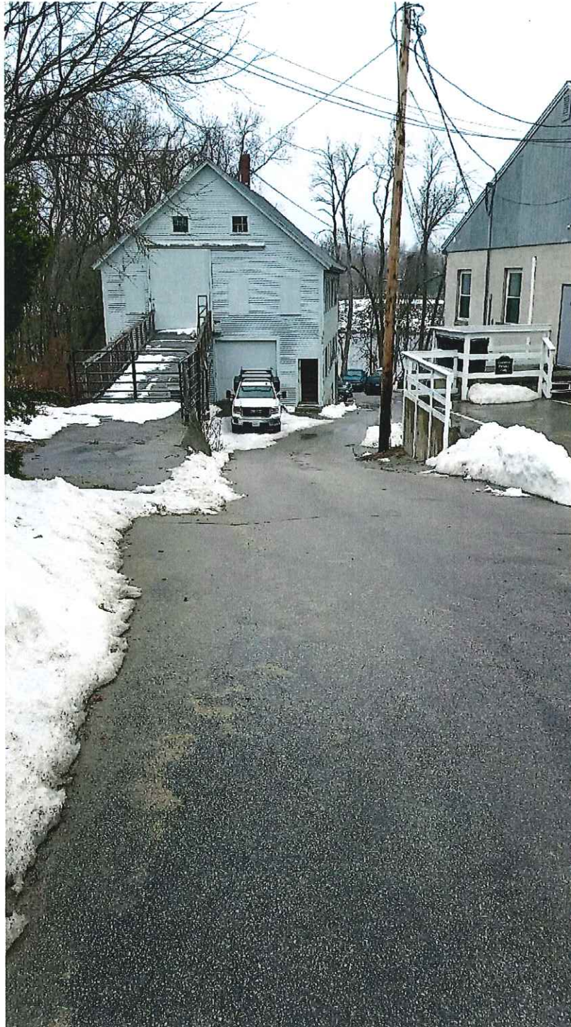
Photo No. 4: Looking west at the existing building to be remodeled (footprint to remain the same), and the existing driveway to be regraded/repaved.
