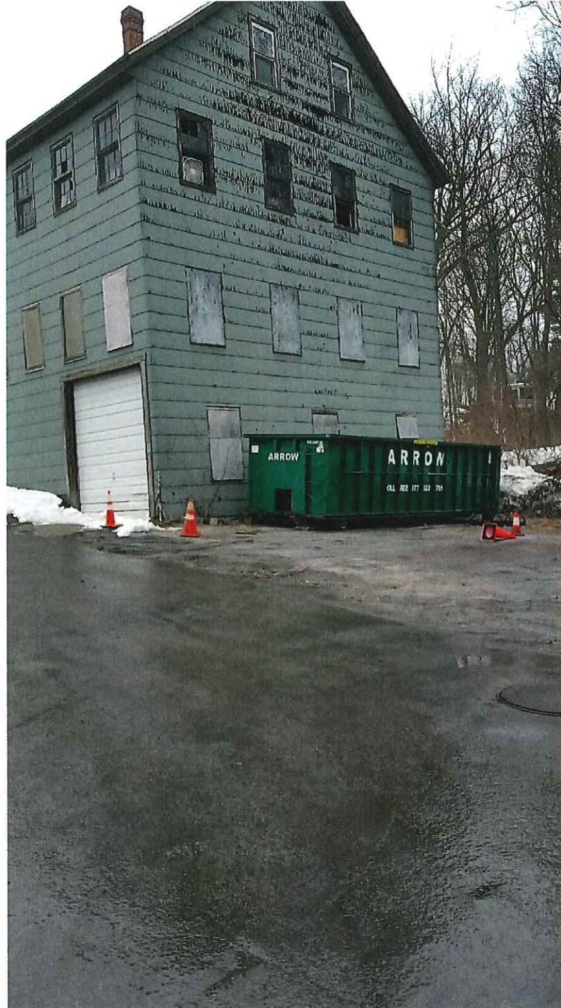
Photo No. 3: Looking east at the existing building to be remodeled (footprint to remain the same), and the existing gravel area to be removed and re-vegetated.
