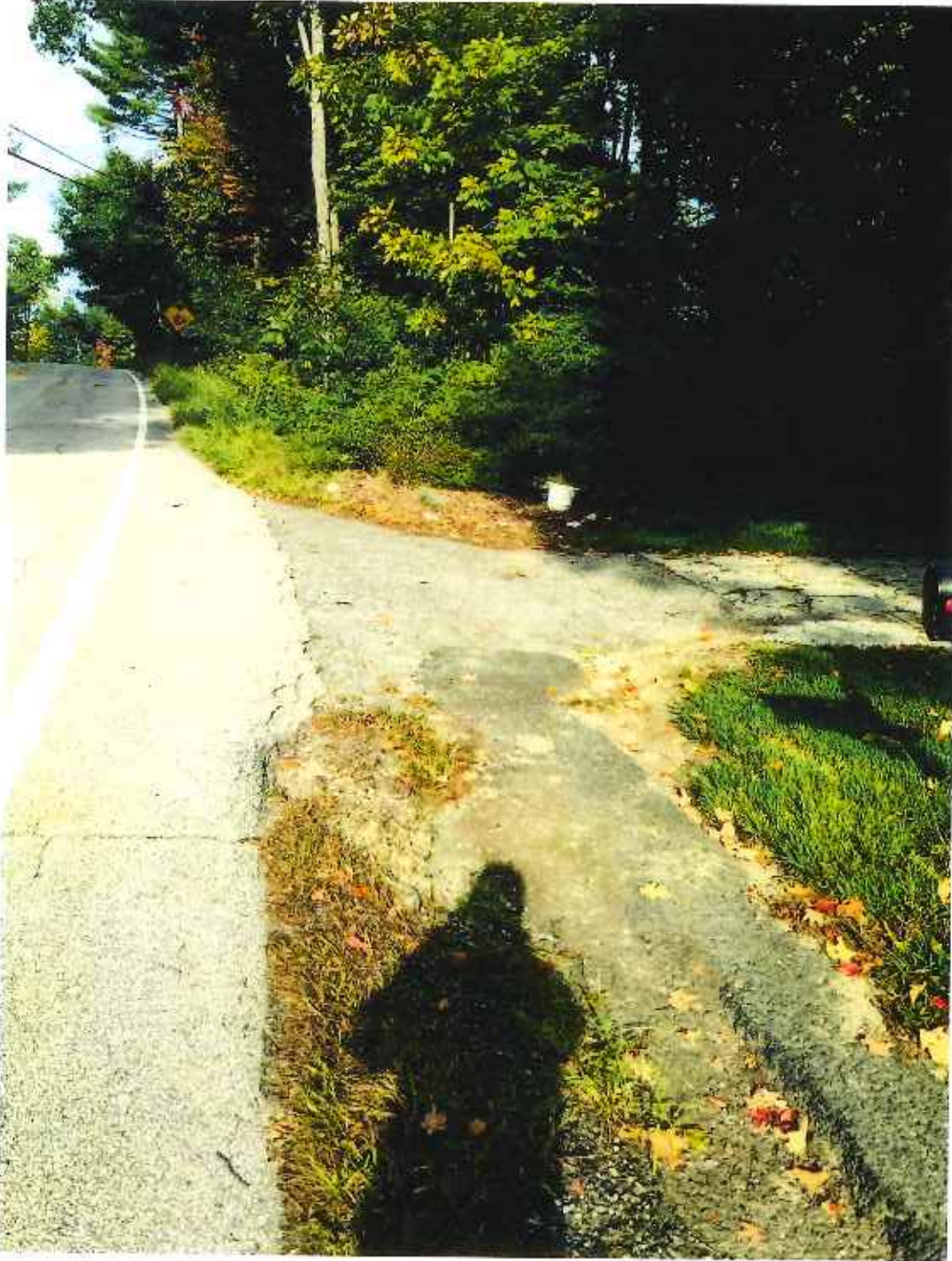
Photo No. 3: Existing driveway to receive roadside ditch culvert.
