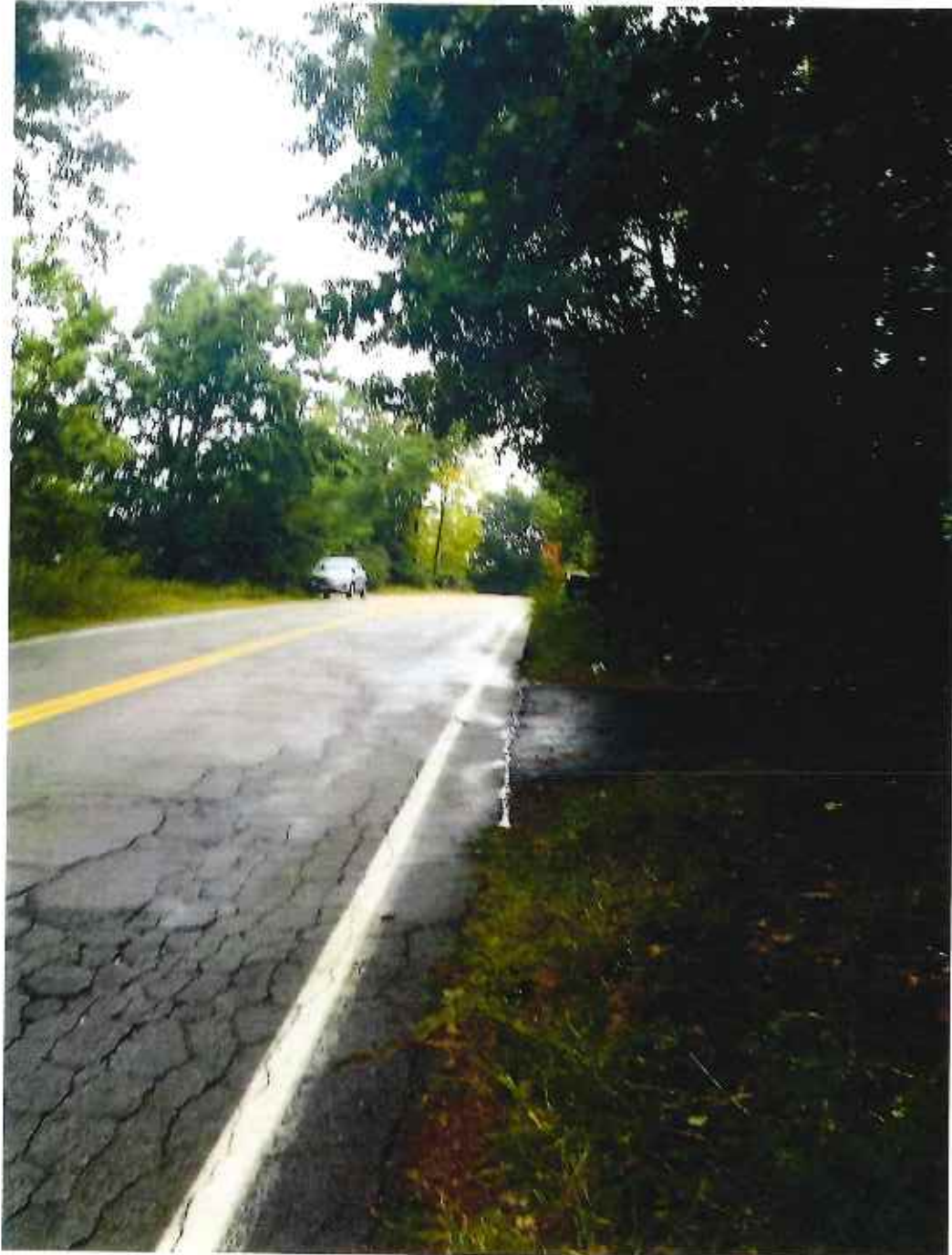
Photo No. 1: Looking right, from the location of the proposed driveway, along Pelham Road.
