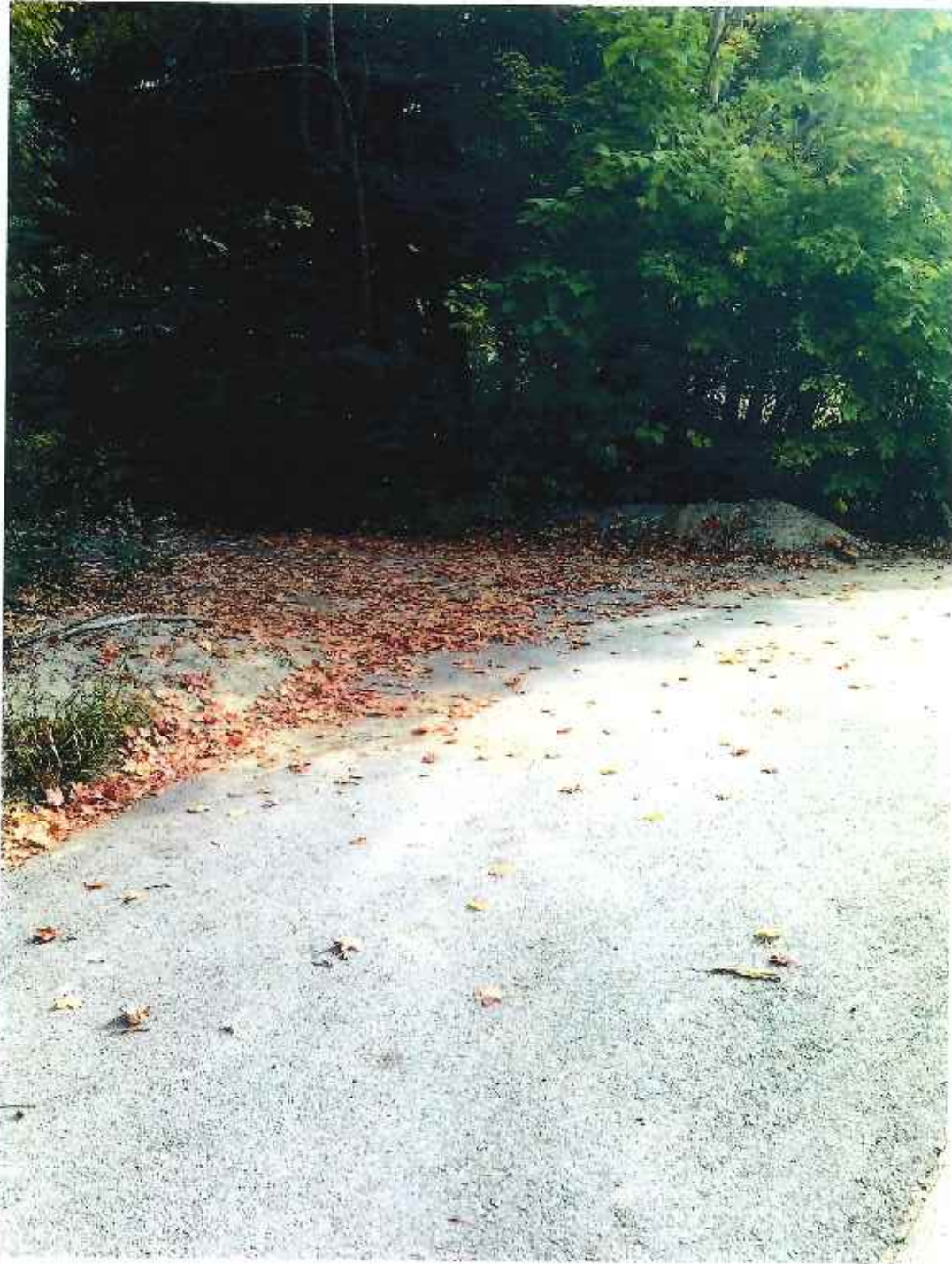
Photo No. 4: Existing driveway to receive roadside ditch culvert.
