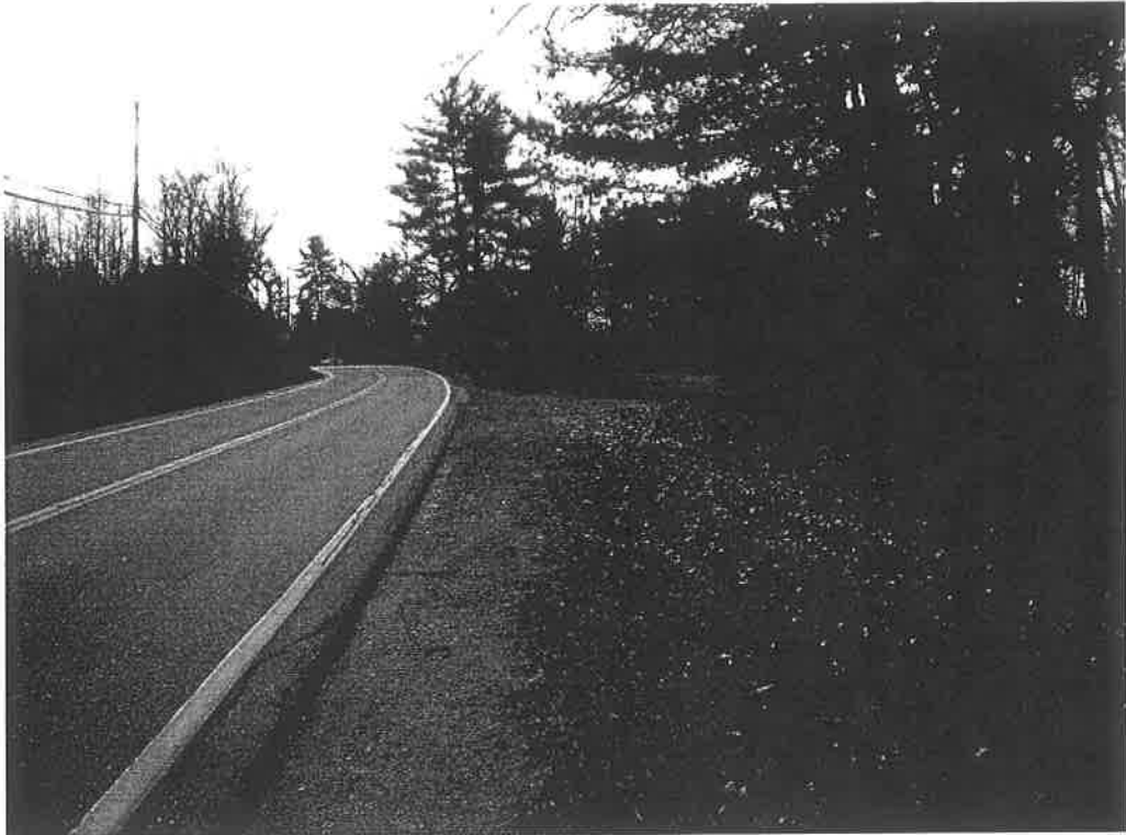
Photo #3 – Webster Street and Lot 6 along the water main route.
