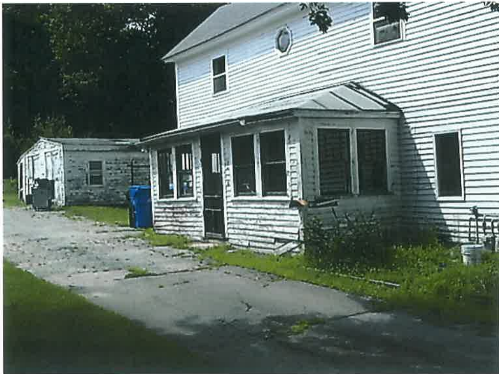
Photo No. 2: The existing two-story wood frame house.
