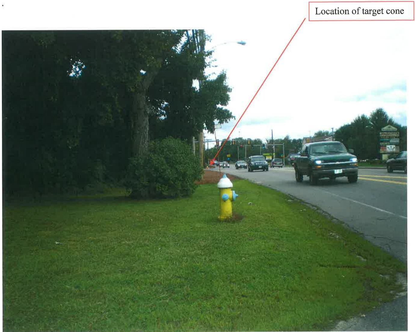
Photo No. 5: Sight distance looking north along Lowell Road toward a traffic cone, placed 400' away.
