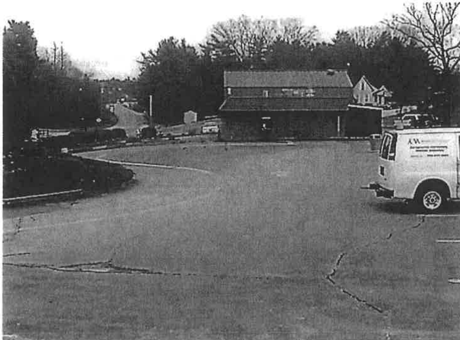
Photo No. 4: Looking east from Adelaide Street toward the site.
