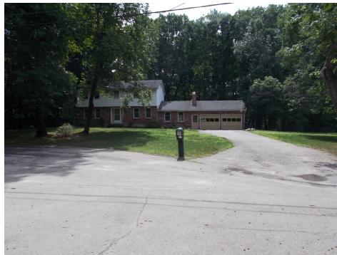
Typical dwelling on Eagle Drive
