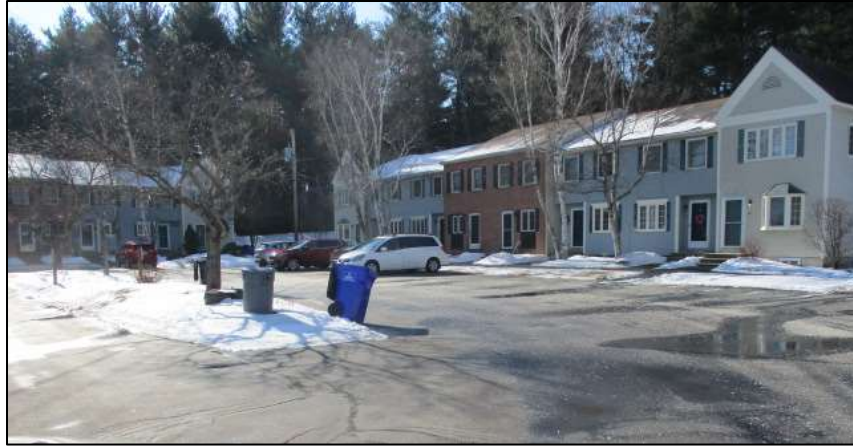
Fox Hollow Condominiums Abutting Subject Property
