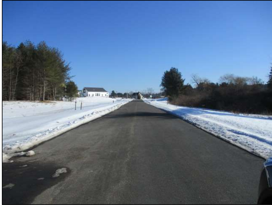
Looking East on Friars Drive Towards Lowell Road
