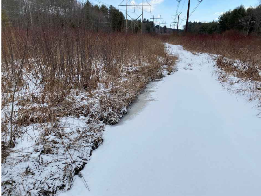
Photograph No. 5: Looking northwesterly at proposed access route associated with Wetland HW-81 and Structure 152 of the 326 Line to be replaced. Timber matting will be used in the wetland portion of the access route.
