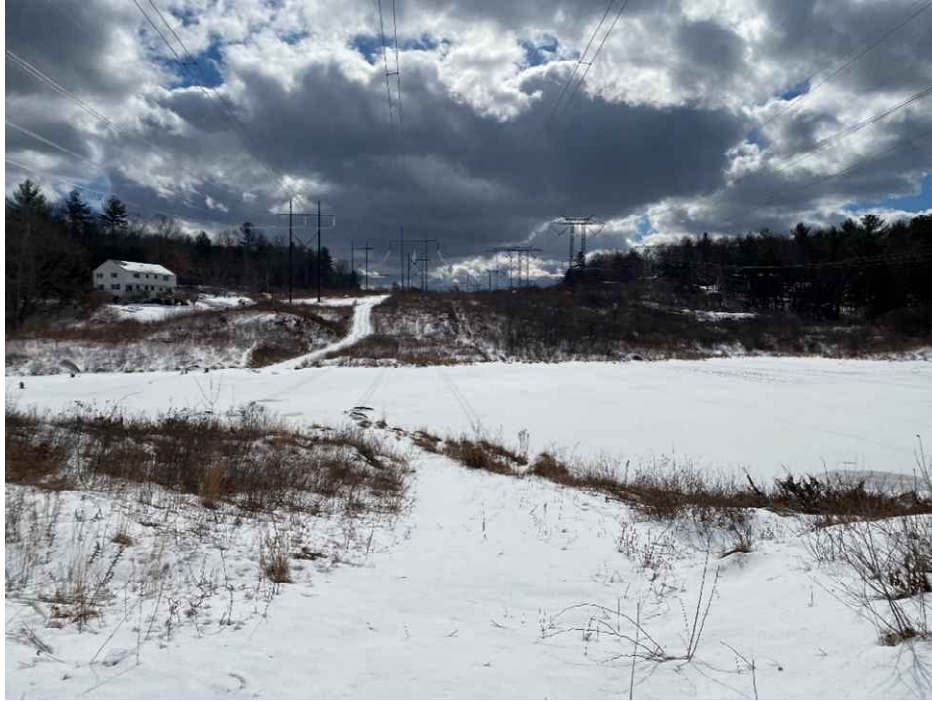
Photograph No. 1: Looking northwesterly at proposed access across Wetland HW-5.1 towards Structure 80 of the 326 Line to be replaced. Timber matting will be used in the wetland portion of the access route.
