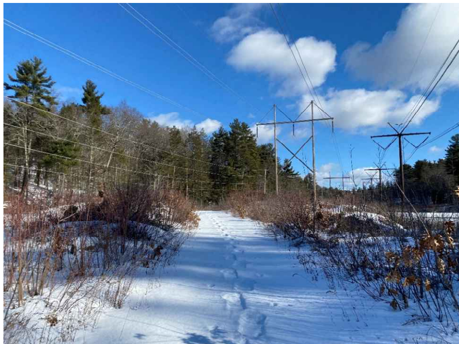
Photograph No. 2: Looking northeasterly at proposed access route to Structure 123 of the 326 Line to be replaced, associated with Wetland HW-45. Timber matting will be used in the wetland portion of the access route.
