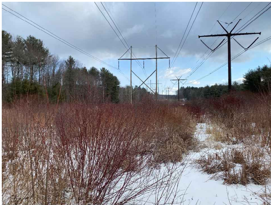
Photograph No. 6: Looking northeasterly at proposed access route and work pad associated with Wetland HW-81 towards Structure 152 of the 326 Line to be replaced. Timber matting will be used in the wetland portion of the access route and work pad.
