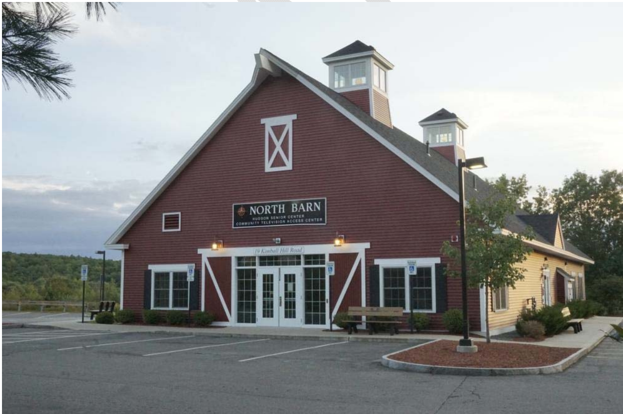
Hudson Senior Center at Benson Park
