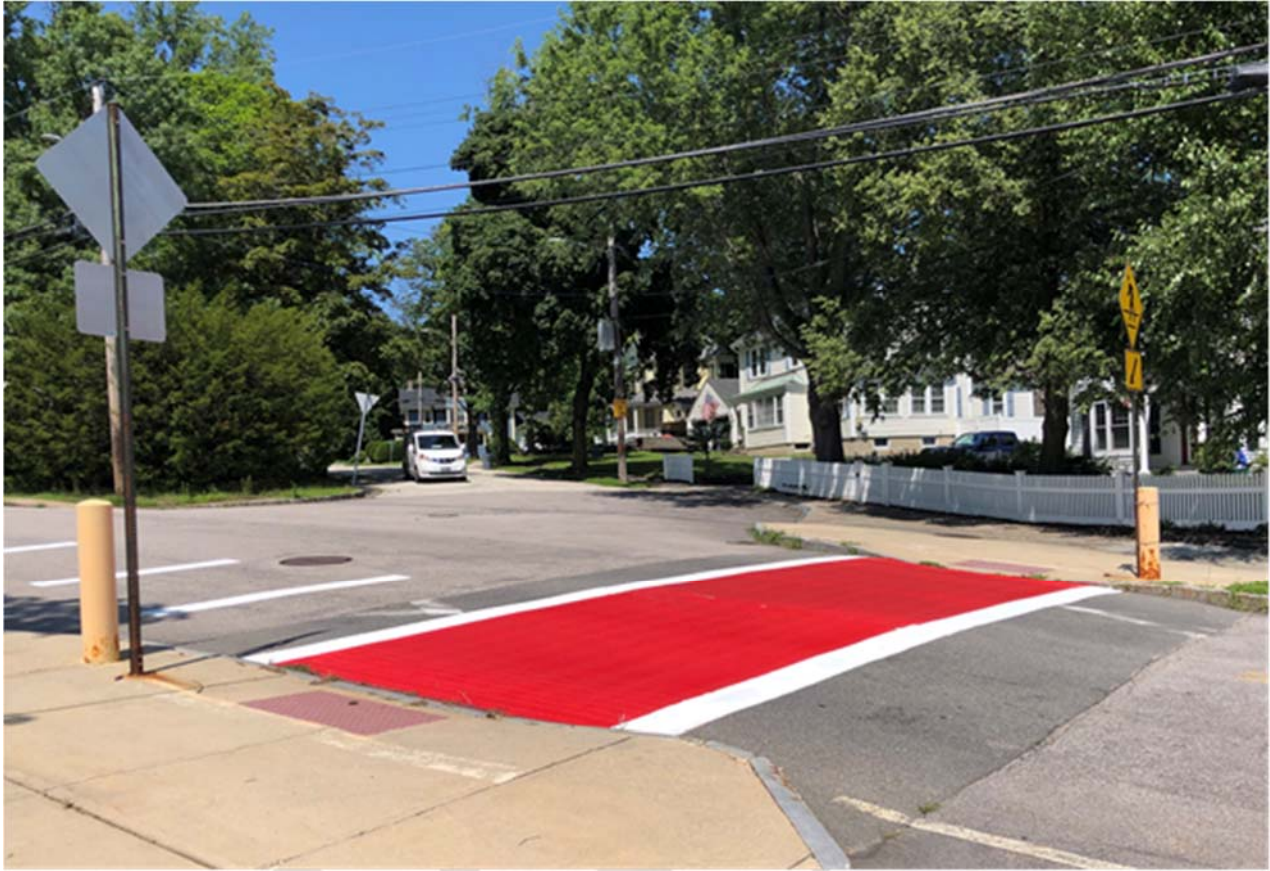
Raised Crosswalk in Nashua
