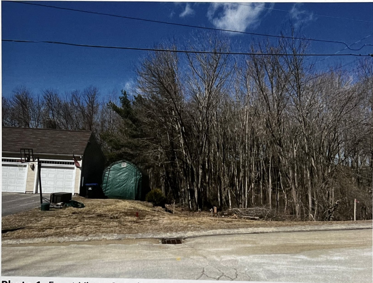
Photo 1: Front View- Standing on Nathaniel Drive, facing the proposed garage, looking north.
