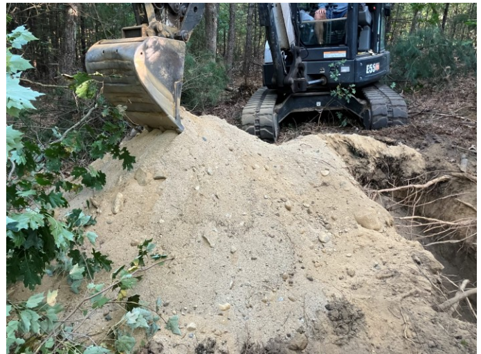
9-16-2024: Test Pit 1 spoils
