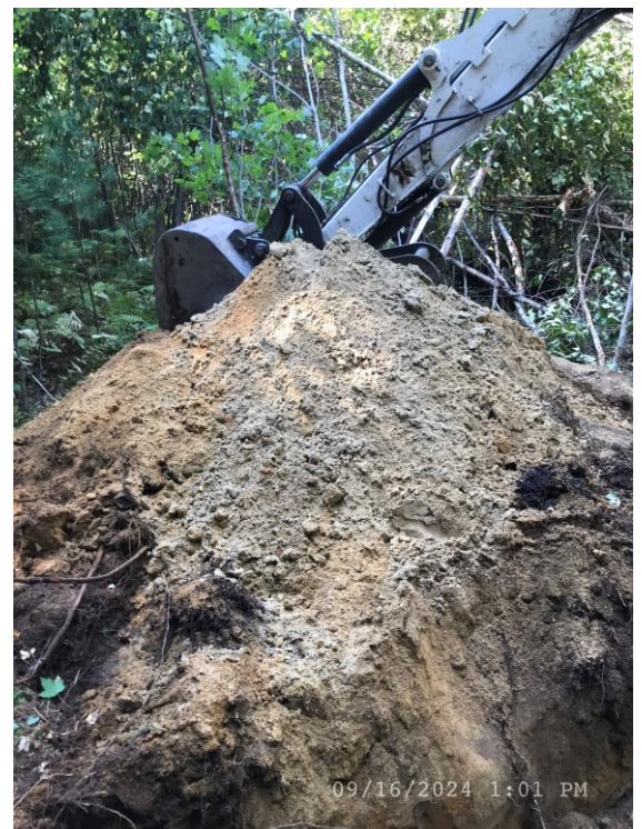
9-16-2024: Test Pit 7 spoil pile
