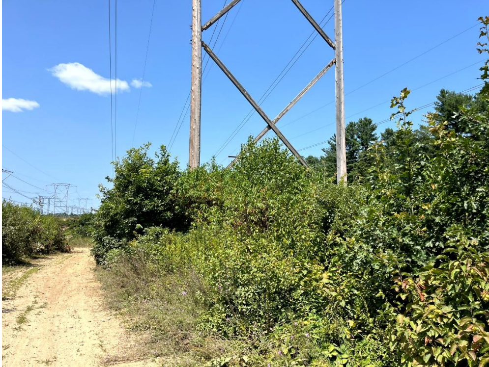
Photograph No. 1: Looking northwest at the proposed work pad location for Structure 74 off Boyd Road, Hudson.
