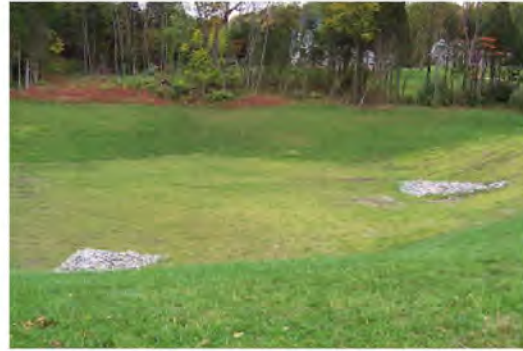
INFILTRATION BASIN WITH SEDIMENT FOREBAY
