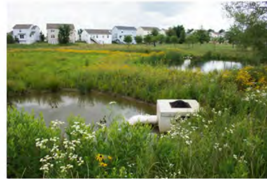
DRY EXTENDED DETENTION BASIN WITH MICROPOL
