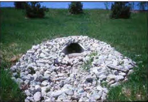
PREFORMED SCOUR HOLES
