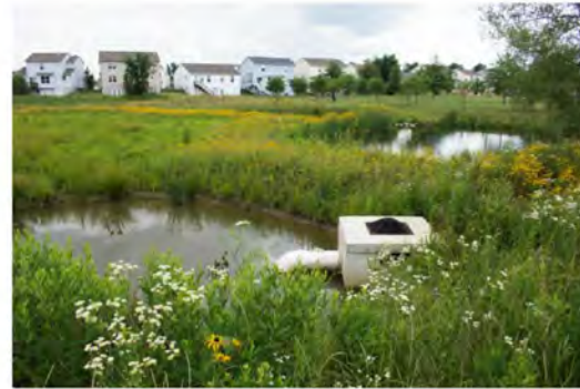
DRY EXTENDED DETENTION BASIN WITH MICROPOL
