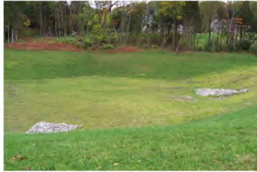
INFILTRATION BASIN WITH SEDIMENT FOREBAY
