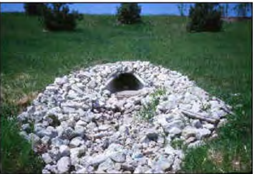
PREFORMED SCOUR HOLES
