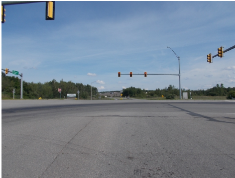
Entrance to Pettengill Commerce Park
