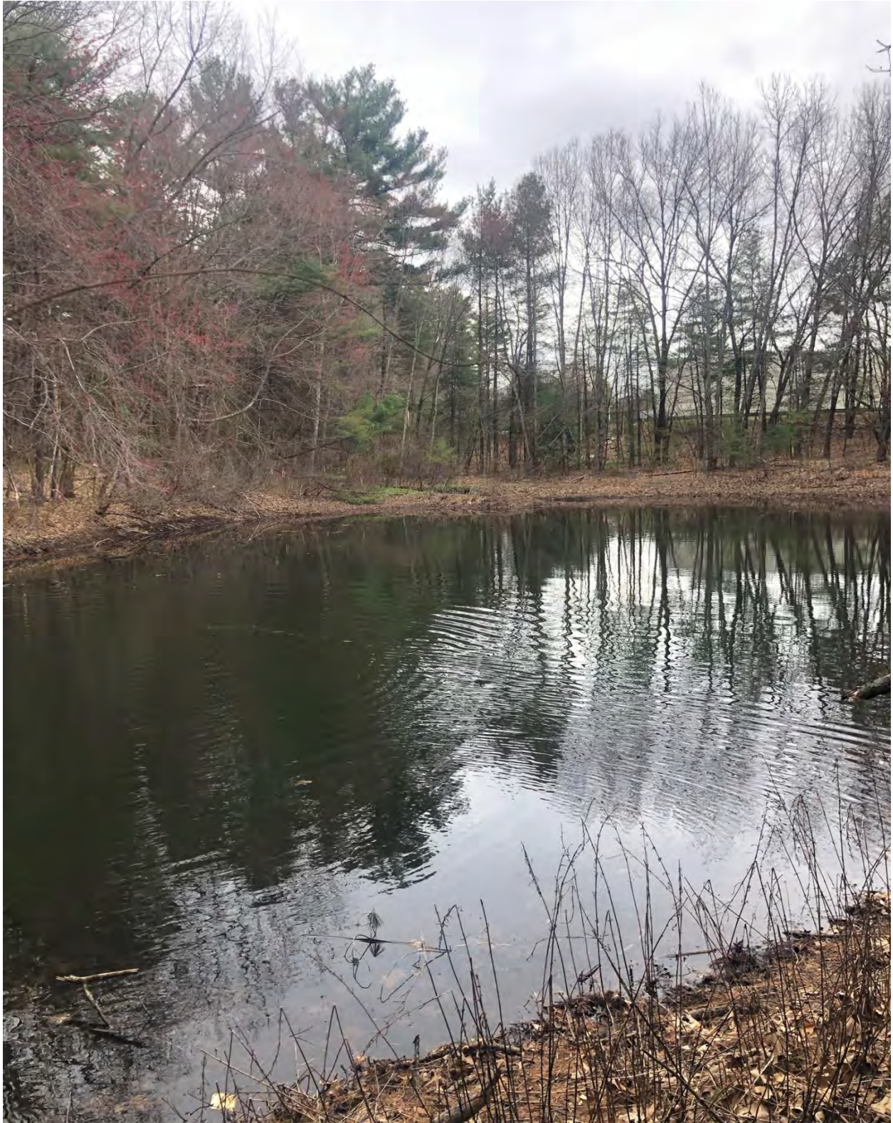
12. View over pond at dam.
