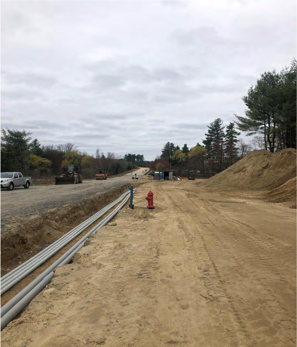
2. Looking west down Friar's Drive, with site on right.
