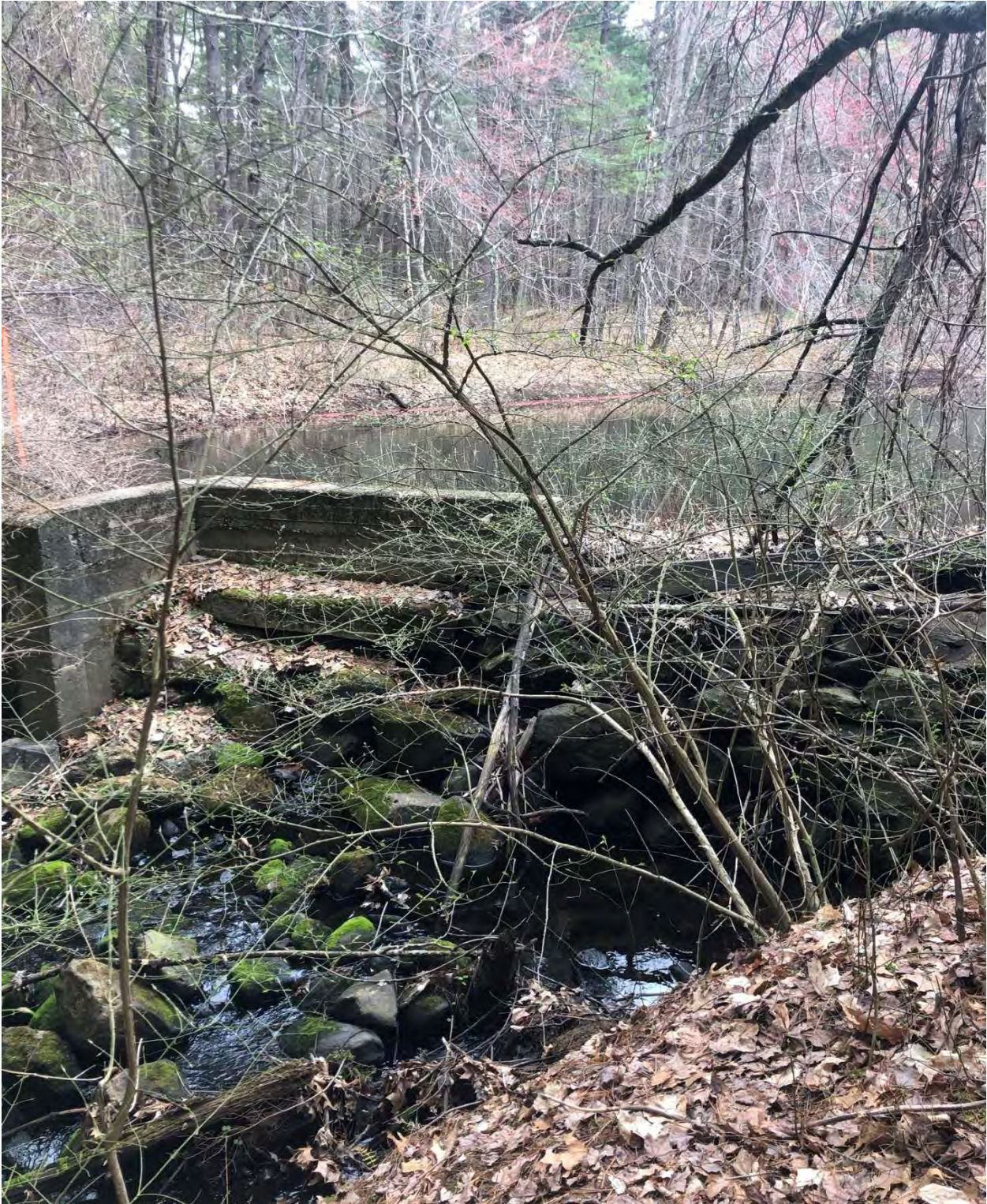
11. View looking east over old dam.
