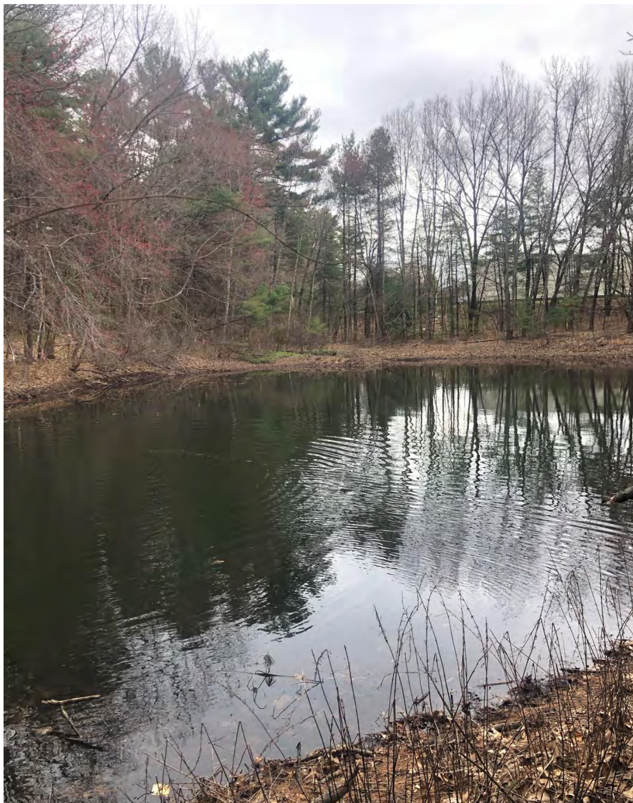
12. View over pond at dam.
