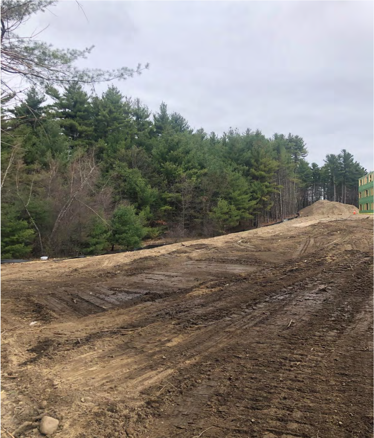
1. Looking west over edge of recent construction project.
