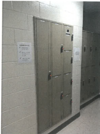
Hudson Police Department Evidence Pass Through Lockers Co-located in Booking/Temporary Detention
