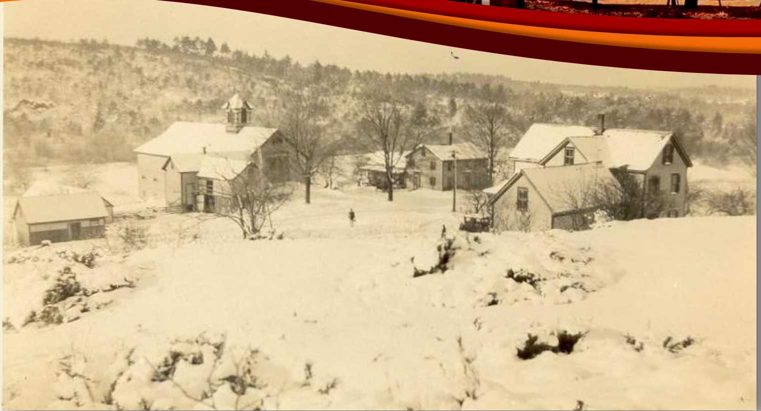
1920 overlooking Haselton Farm from hillside above 25 Bush Hill Road
