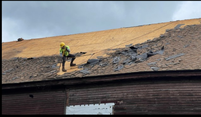
A NEW BARN ROOF Featured Story, pg. 4
