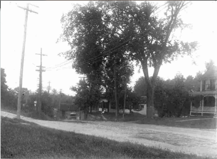
Trestle crossing over Lowell Road south of Central Street
